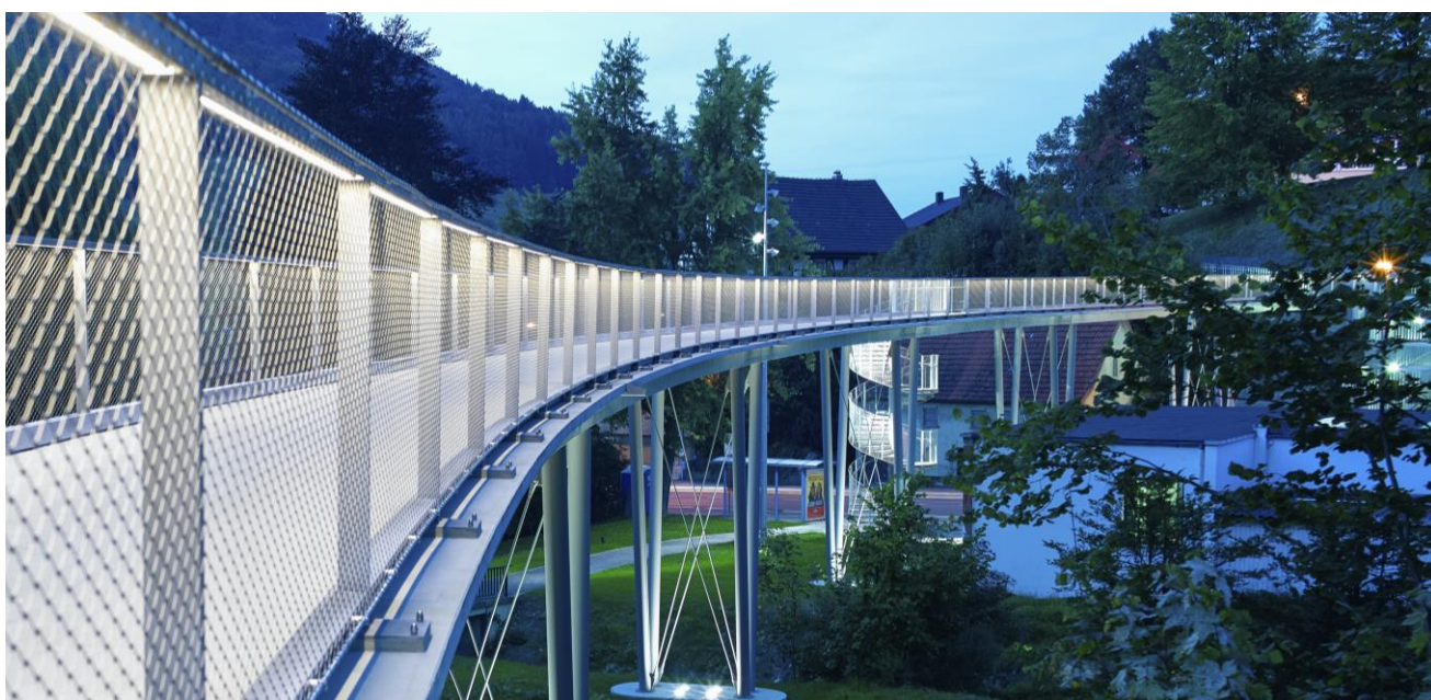
The pedestrian and bicycle bridge in Albstadt, Germany, is an early example of a textile-reinforced concrete structure. The bridge is about 100 meters long. Image: Udo Jandrey
