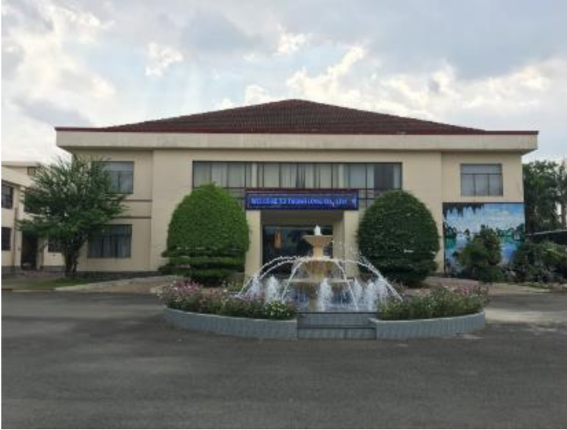
Main building entrance of Vietnam-based Tuong Long, the first denim manufacturer in Vietnam to switch 100% of its production to Archroma's aniline-free* Denisol® Pure Indigo. (Photo: Tuong Long)
